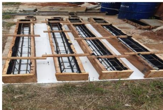
Fig. 4. Wooden formwork for Beams
